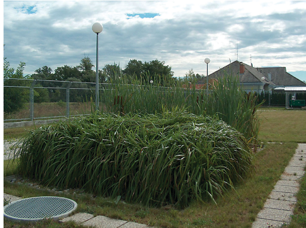
Figure 15: Constructed wetland in location Hrušćica near Zagreb; photo by Renata Horvat.
