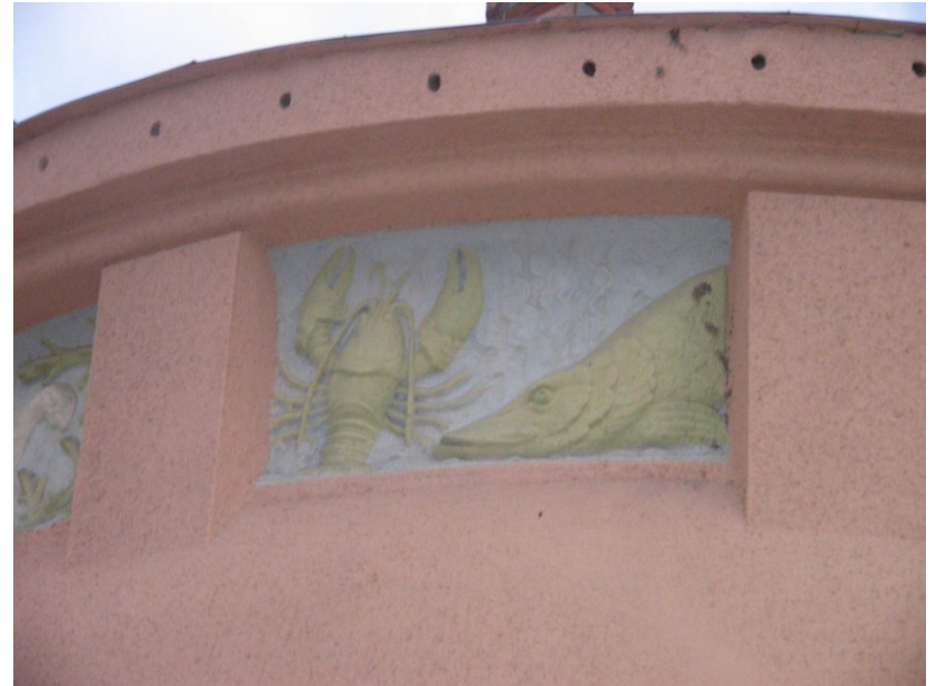
Market building Kuopio, Finland
